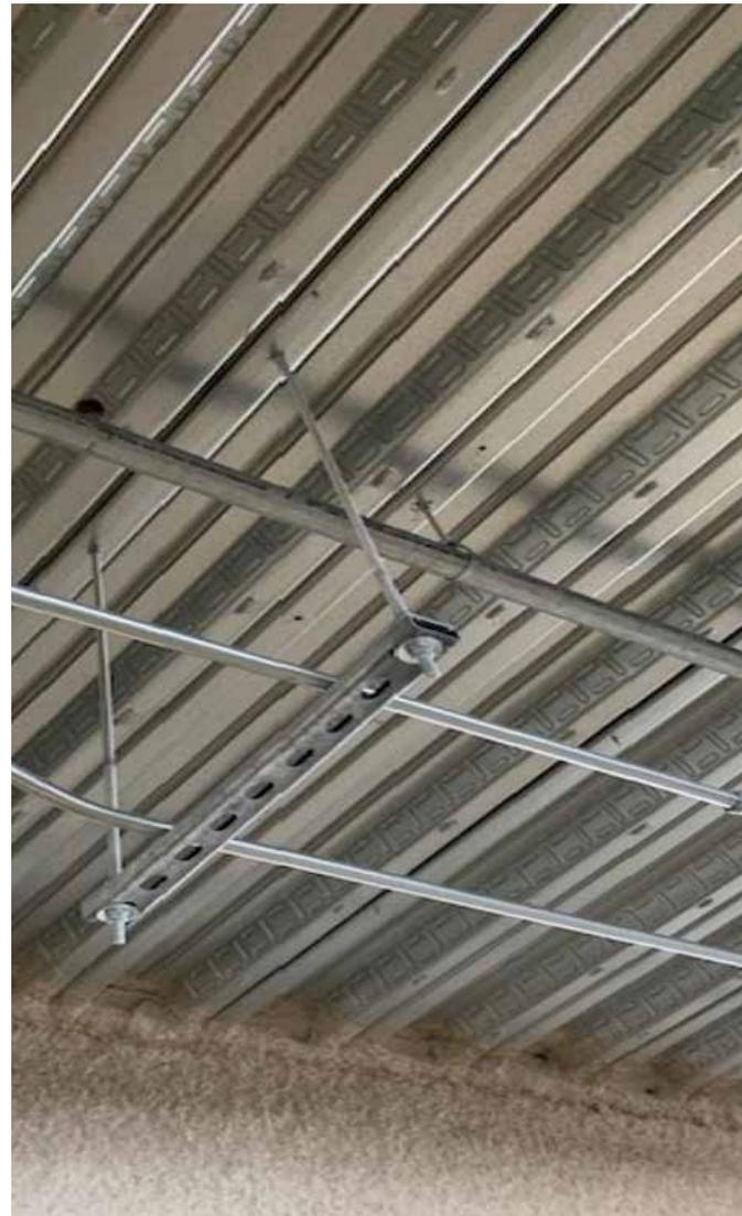
Contractors have long trusted the dependability, effectiveness and convenience of Sammy X-Press – even in challenging conditions. The threaded rod hanging fasteners are a revolutionary product, particularly for awkward and tight spaces. In addition to installing into a variety of steel thicknesses up to 1/8”, the fasteners can accommodate vertical, horizontal, and swivel installations at an angle of up to 89 degrees.
